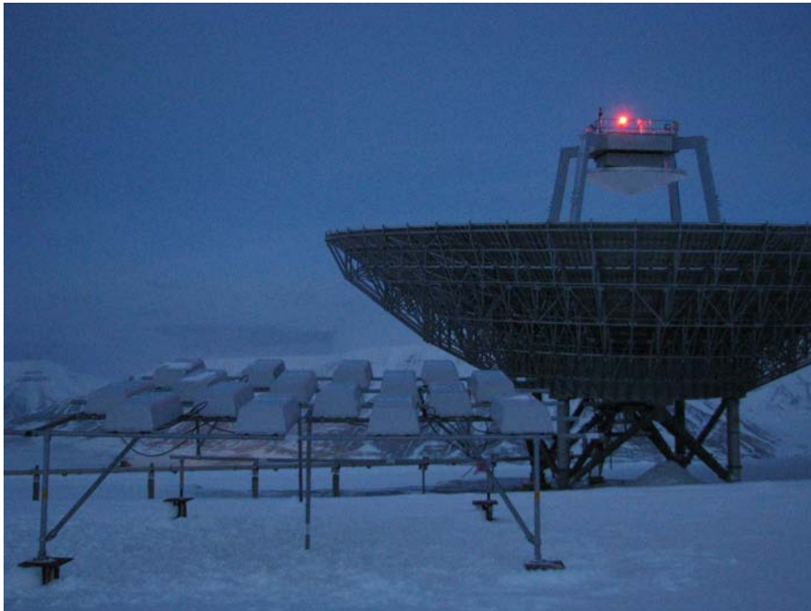
Figure 7.2: Photograph of one of the new panel-antenna arrays, with the ESR 42 m dish in the background, taken by the author during the construction of the interferometry receivers in November 2007
