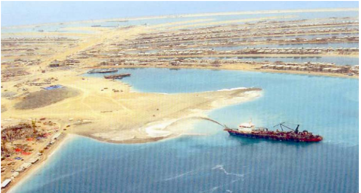
Figure 7.2 Barge Dredging Sand from the Sea Reclamation Stage of JPI in 2004.
