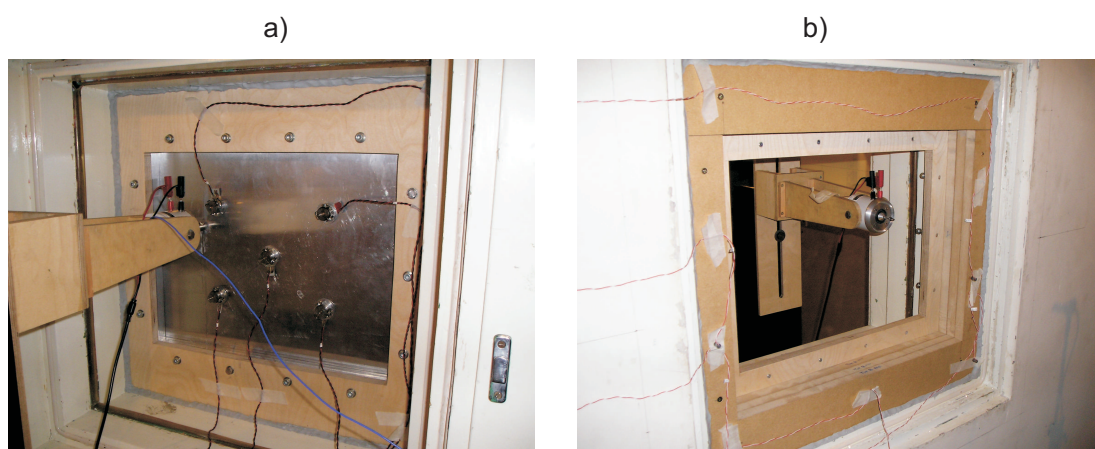
Figure E.7: Pictures of the shaker arrangement on the source side of the panel.
