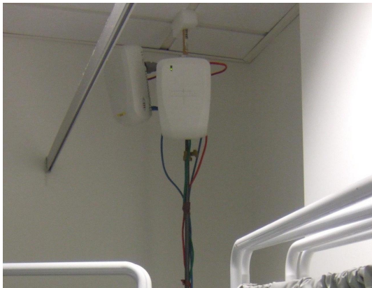
Figure 6. Sensors positioned around the room.
