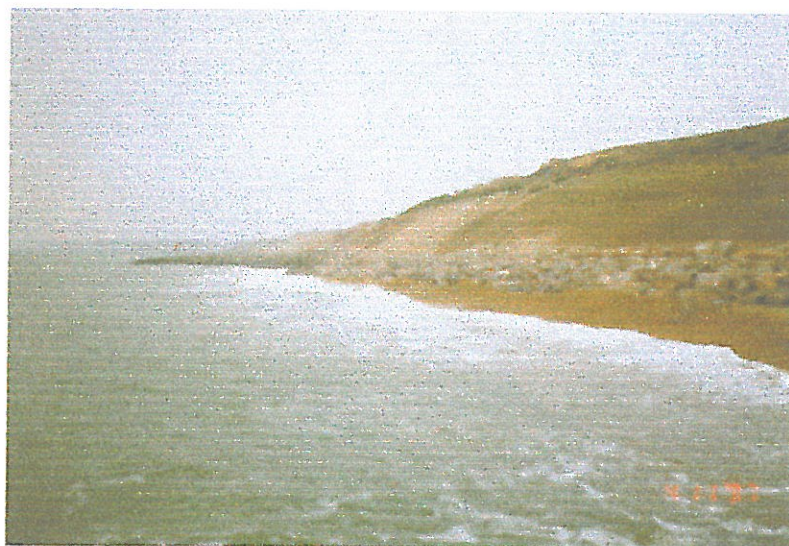
Figure 2 - Rock Armour Protecting the toe of the Cliff from Marine erosion
