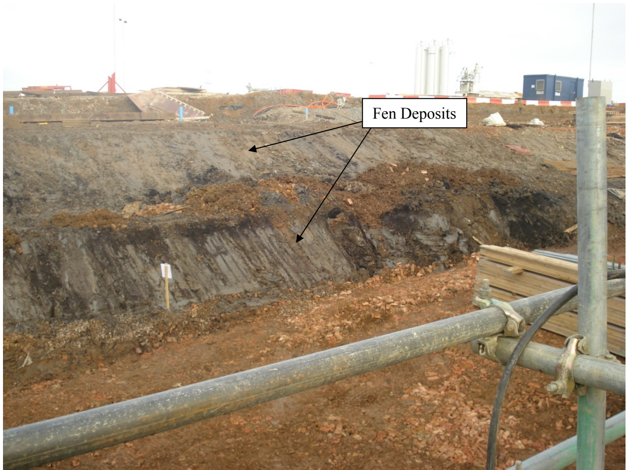
Figure 4-9: Cut in the west slope showing Fen Deposits
