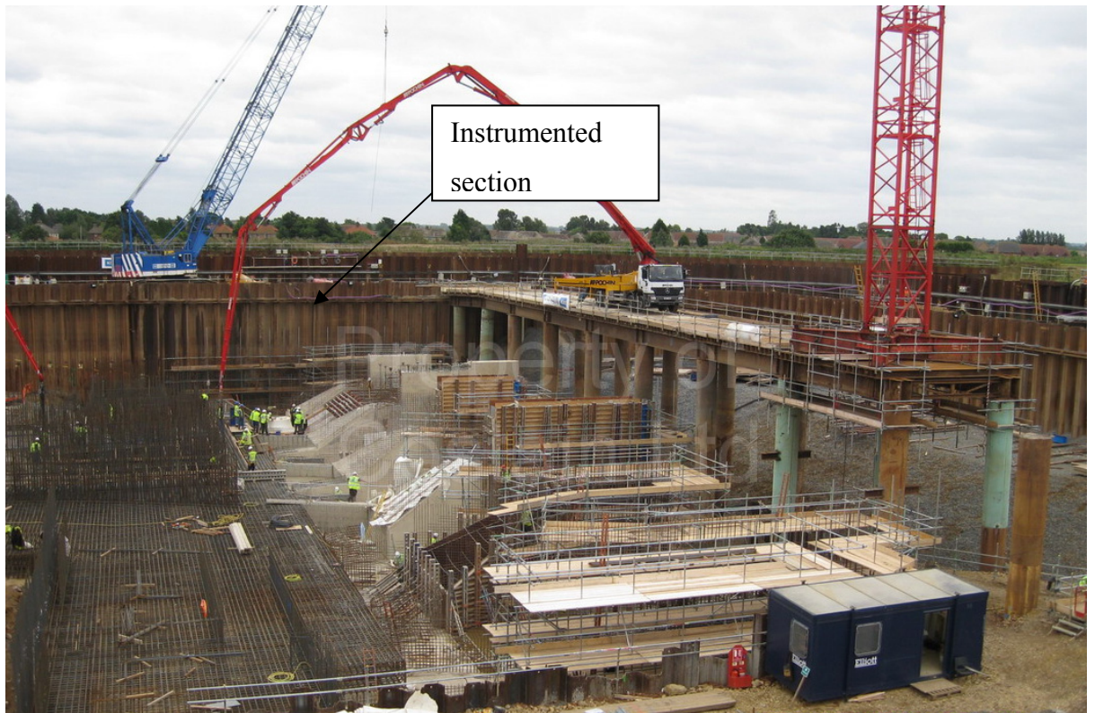
Figure 7-48: Pump base completed (Date 18/08/2008)
