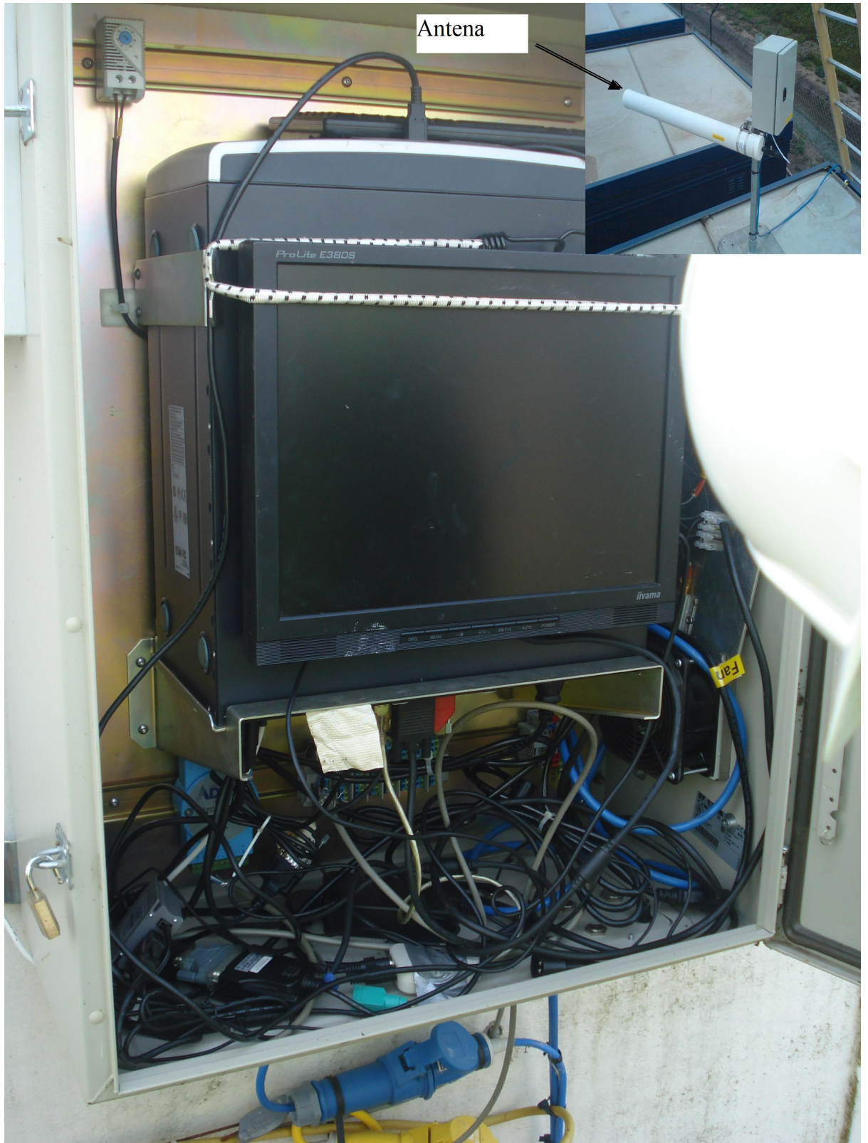
Figure 7-15: Site computer, used for data storage and communication
