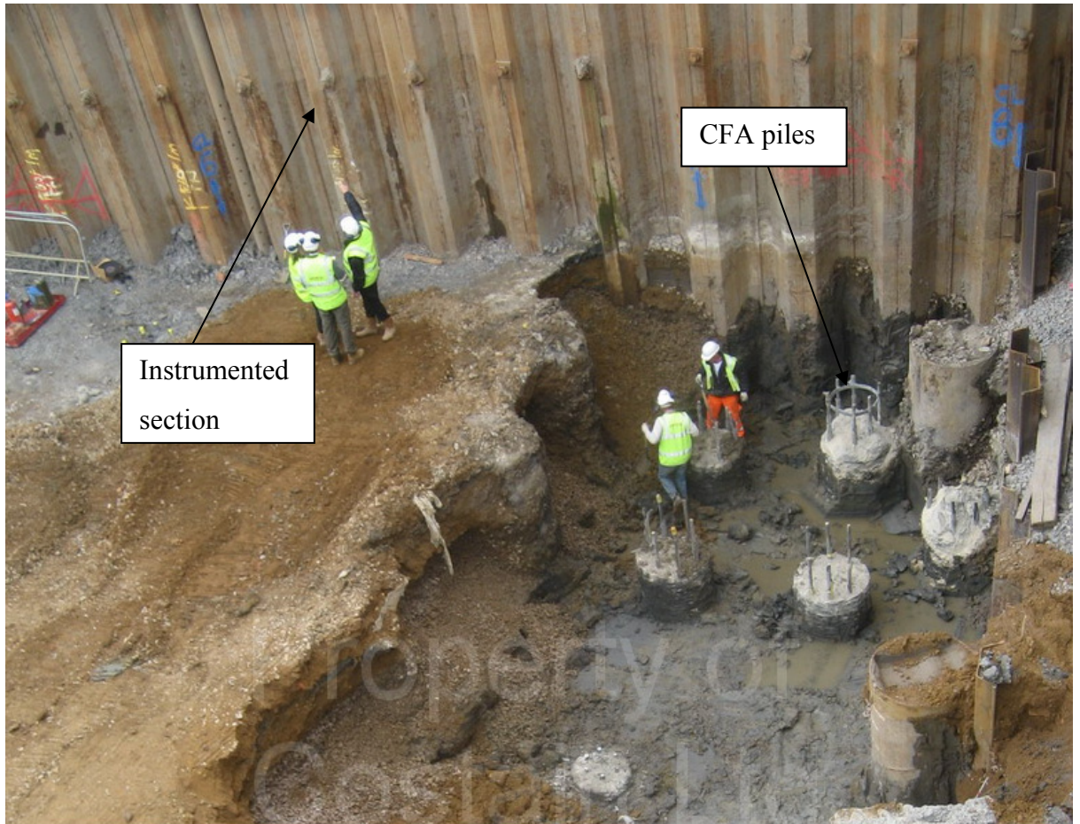
Figure 7-45: Excavation to 92m MLD in front of Cell C3 to facilitate placement of piling mat (16/06/2008)
