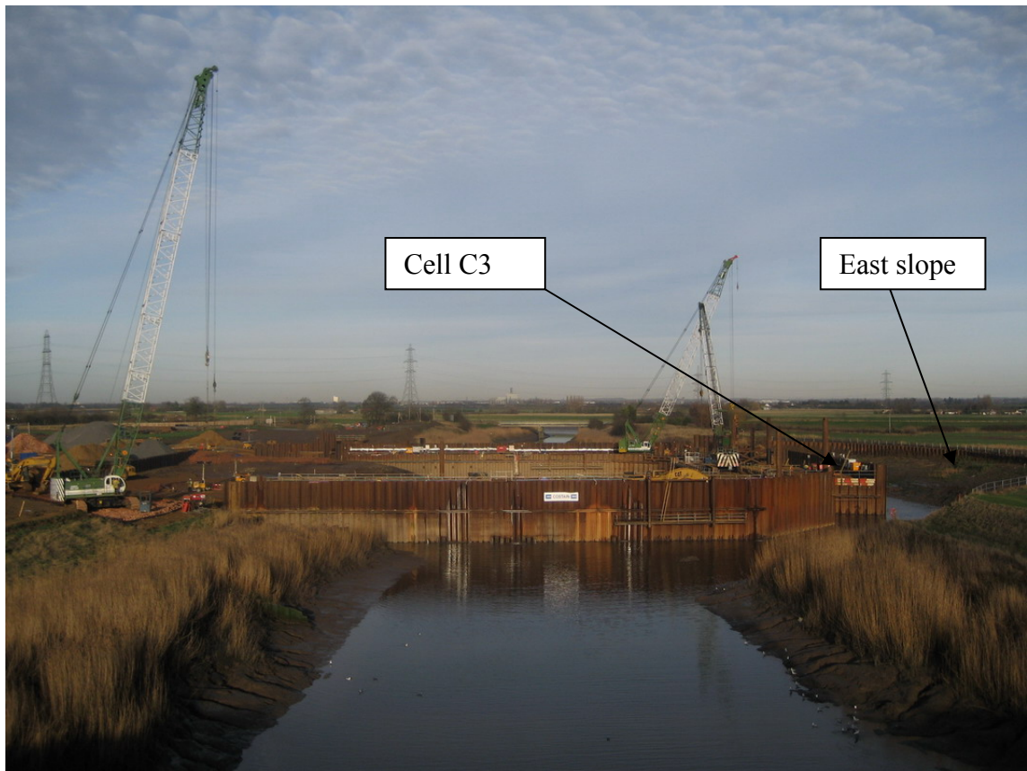
Figure 7-49: East slope and central cells construction
