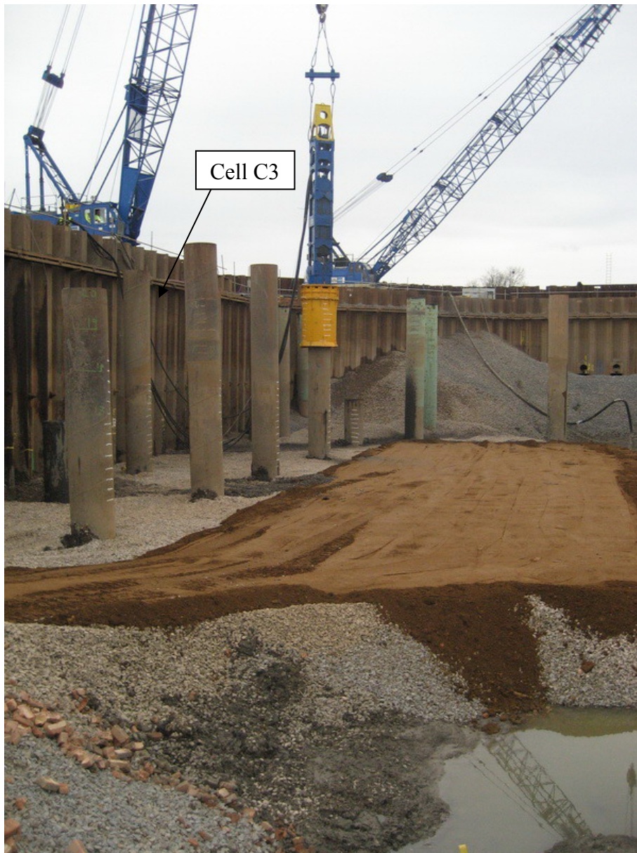
Figure 7-42: Steel pipes used for jetty are hammered in to facilitate installation CFA piles once the jetty was removed (25/04/2008)
