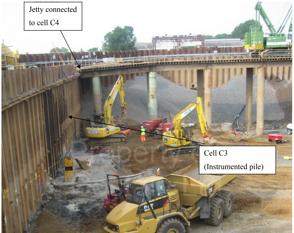
Figure 7-44: Front jetty connected to walling beam on cell C4 (12/06/2008)
