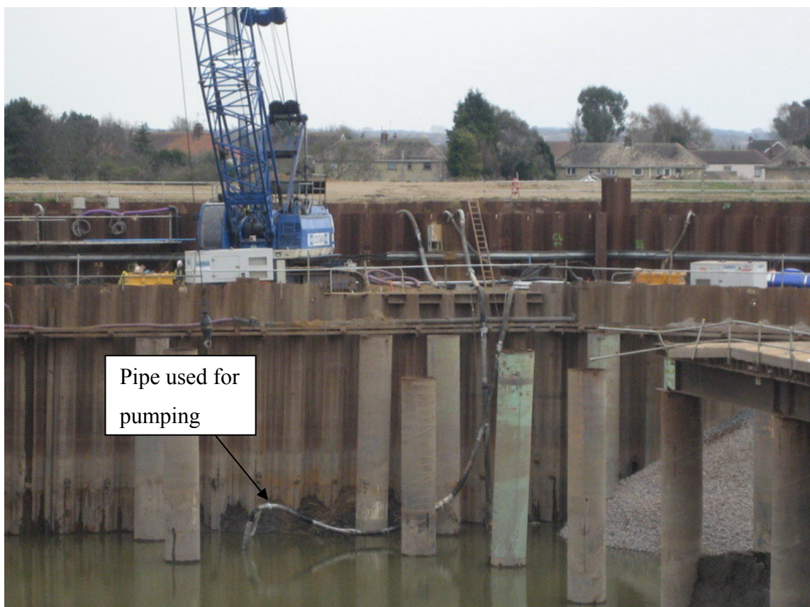
Figure 7-40: Water being pumped out of the cofferdam enclosure (10/04/2008)
