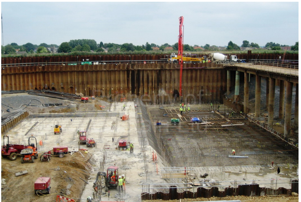
Figure 7-47: Base slab poured (Date 15/07/2008)
