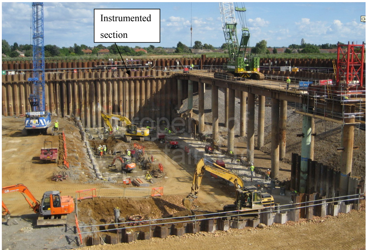
Figure 7-46: Piling mat completed in front of cell C3 (Date 03/07/2008)
