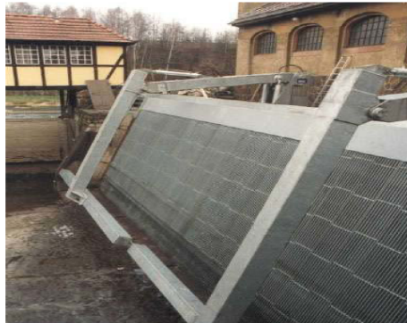
Figure 2.8: Raked bar screen (Bacon 2004)
