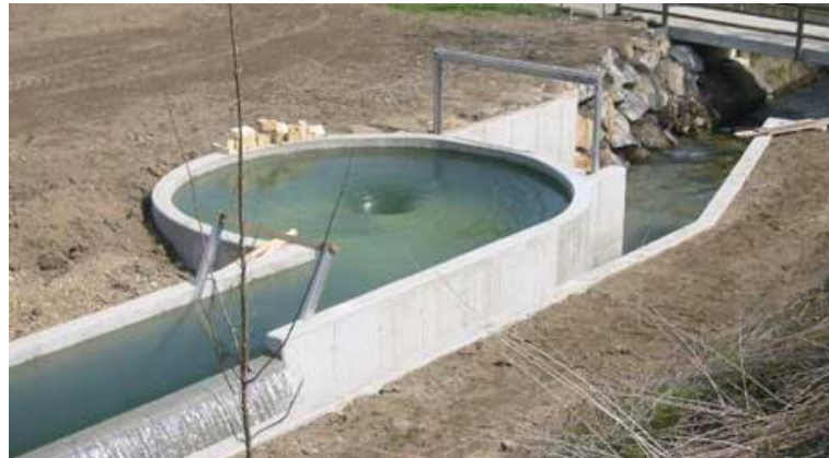
Figure 3.27: Gravitational Vortex Machine prototype (Zotlöterer 2006)
