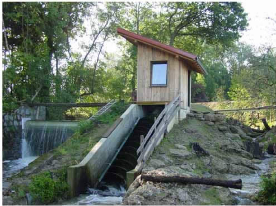
Figure 3.17: Archimedes Screw installation (Atro 2006)
