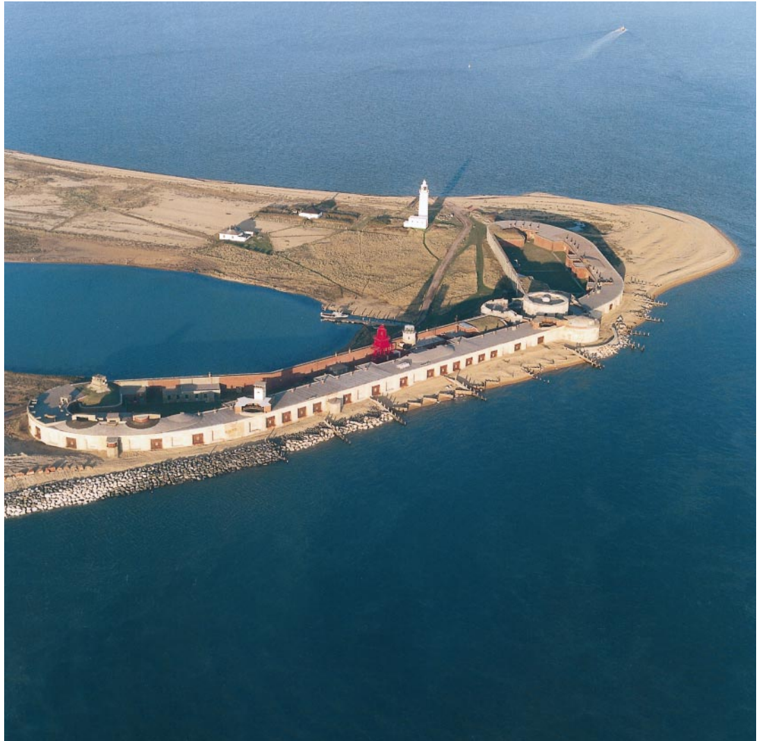
Fig. 7. Hurst Castle at the end of the stabilized spit
