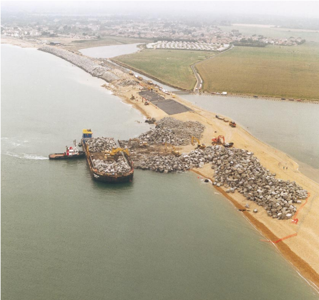
Fig. 6. Use of two rock delivery barges ensure completion before winter storms
