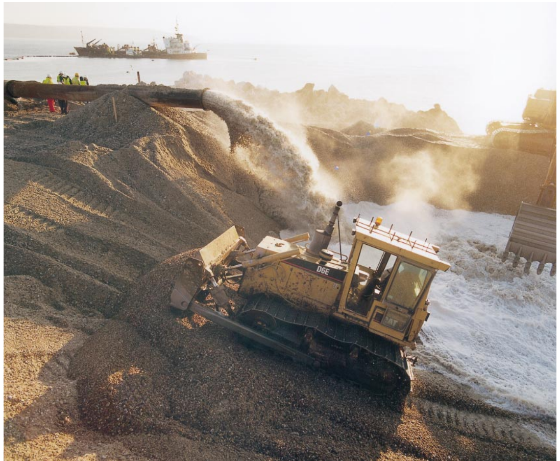
Fig. 4. Marine gravel being pumped on to spit
