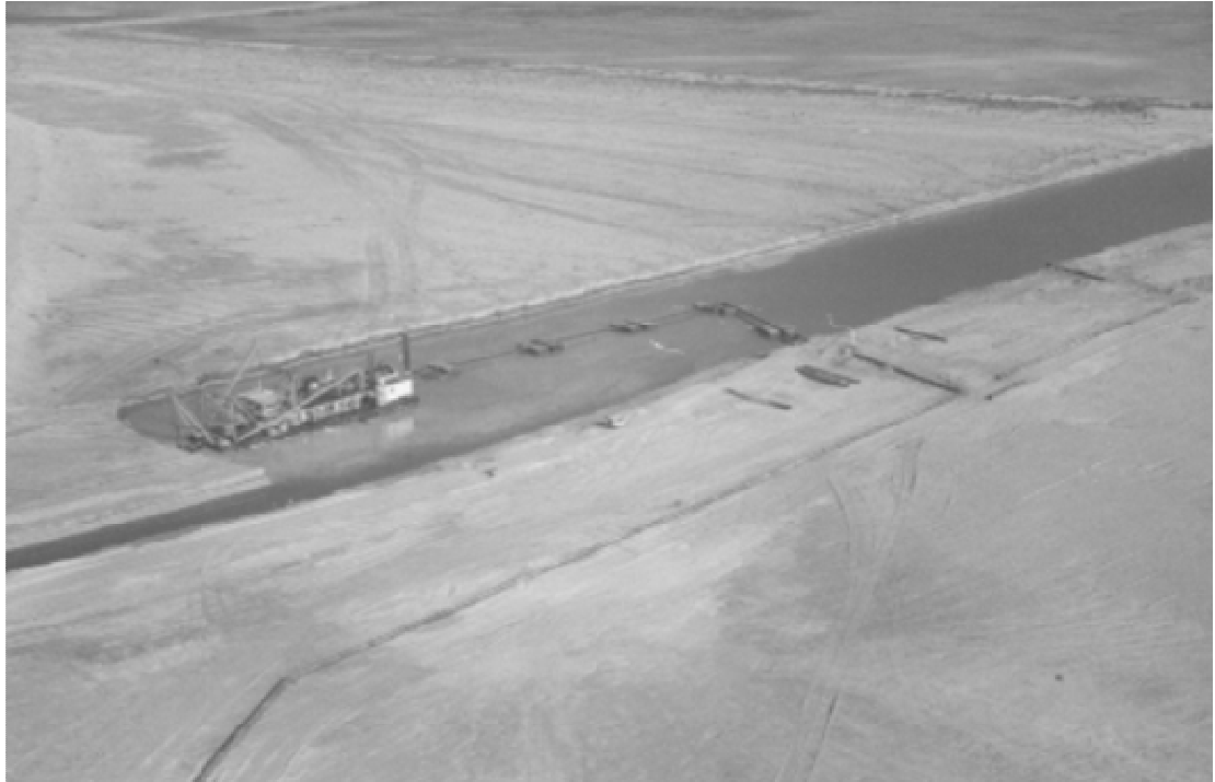
Figure 2.4 Single cut dredging project (Courtesy Gulf Cobla L.L.C.).
